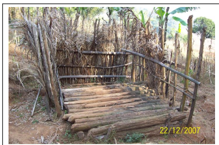
State of latrine before construction
