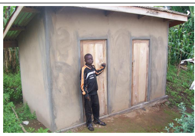
Built latrine and wash room
