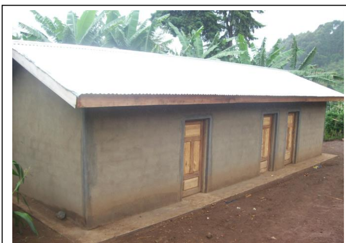
House after rehabilitation
