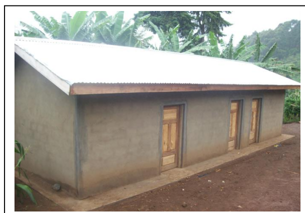
House after rehabilitation
